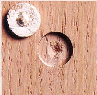
Excessive shrinkage led to adhesion problems with this powdered putty.
